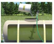
Gel System: Gel crystals are added through vent pipes before injection.
